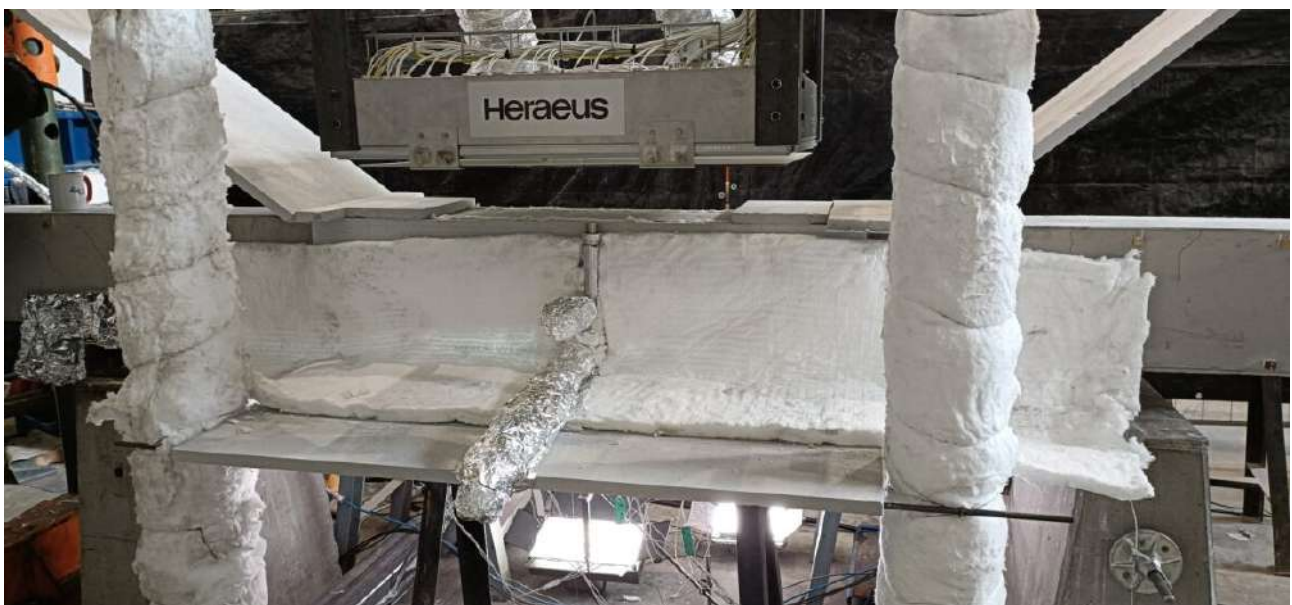
Figure 3. Insulation protection on the beams
