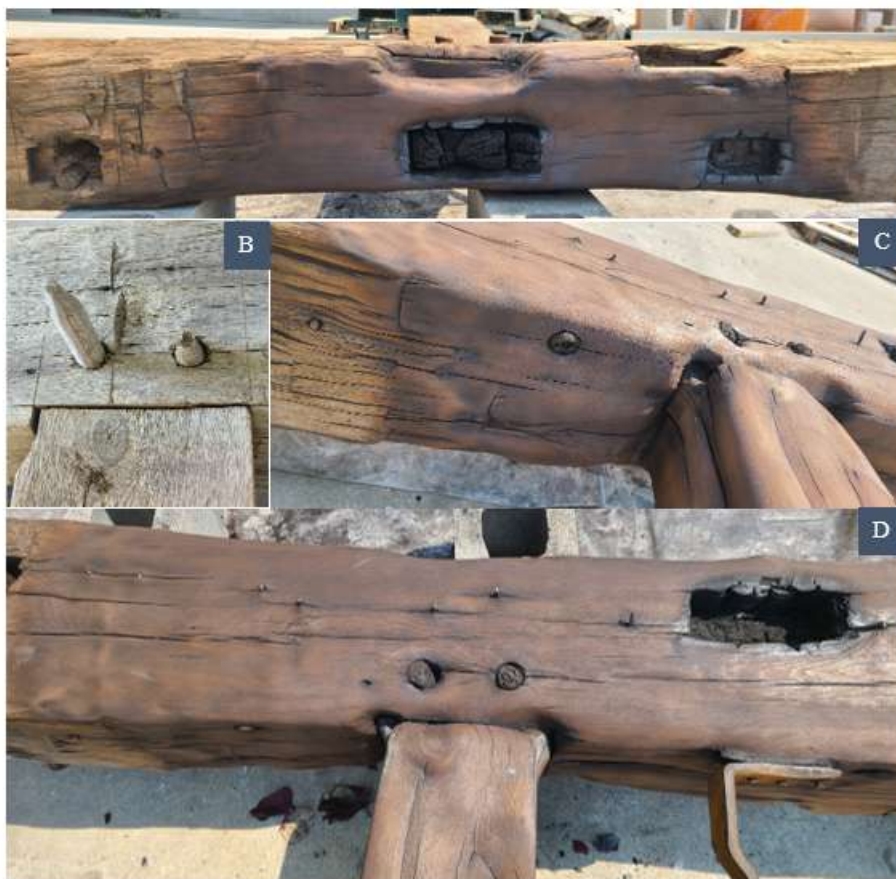
Figure 9. Connector after Char Removal
