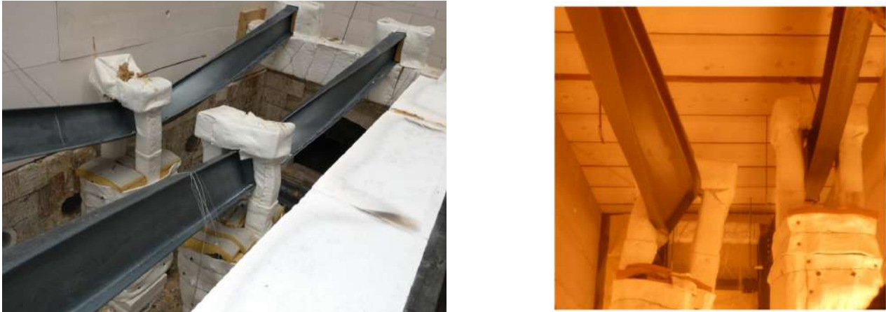
Figure 8. Test specimen during and after the fire test
