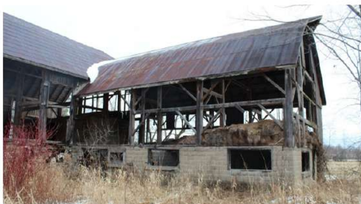
Figure 3. Heritage farmstead structure dating to early 1800s (Author's photo)
