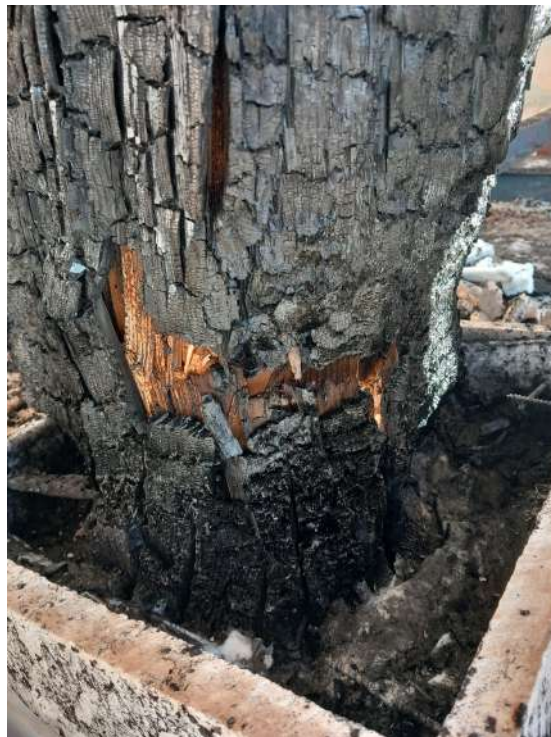
Figure 7. Foot of the column of Test 20 after the test
